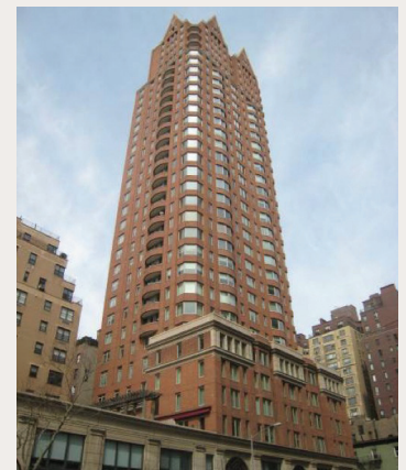
Figure 4: Aluminum punch windows and brick cladding (New York, NY)
