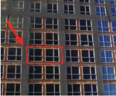
Figure 14, 15 and 16: Identification of representative areas for field testing (precast concrete/punch window wall assembly)
