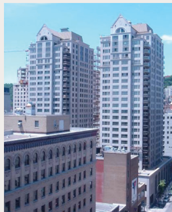
Figure 3: Aluminum punch windows and precast concrete (Montreal, QC)
