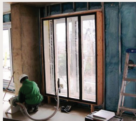
Figure 21: Interior test chamber used to test a punch window assembly
