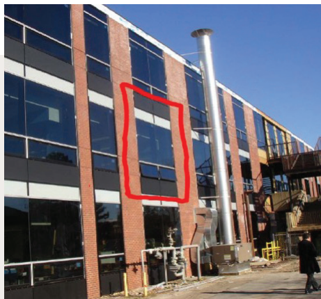
Figure 18: Identification of representative area for field testing (metal and glass curtain wall and adjacent masonry assembly)
