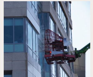
Figure 24: Dynamic water penetration field test as per AAMA 501.1
