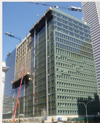
Figure 2: Metal and glass curtain wall - building reclad (Montreal, Quebec, Canada)
