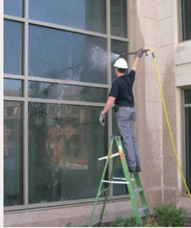
Figure 33: Diagnostic hose testing of curtain wall section
