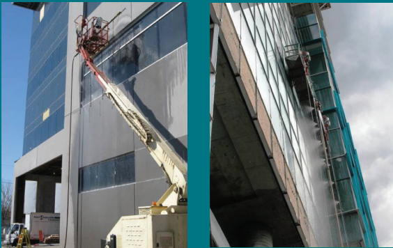
Figure 12 and 13: Field testing for resistance to water penetration
