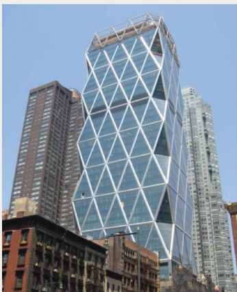
Figure 1: Metal and glass curtain wall - new construction (New York City, New York, USA)
