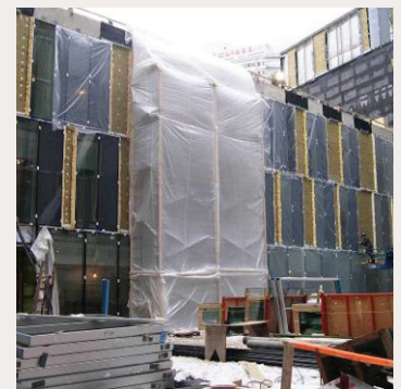
Figure 32: Temporary exterior heating via test specimen
