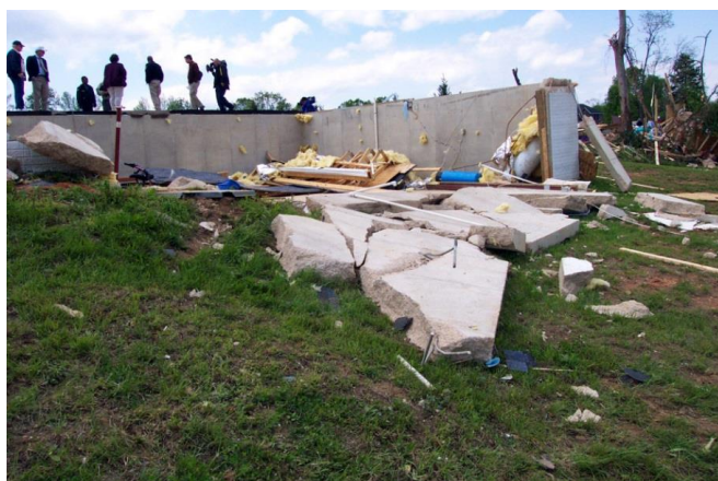
Tornado damage to home in La Plata, Md., taken April 29, 2002, a day after a deadly tornado outbreak. Photo courtesy of NOAA.
