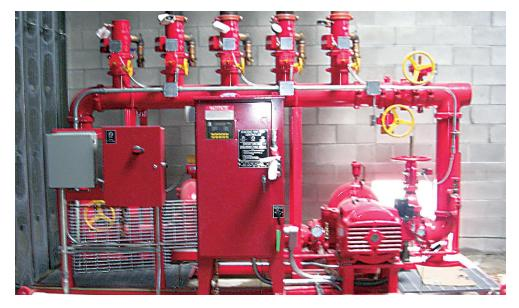
Fire pump controllers are control panels containing electrical components such as circuit breaker, switches, relays and other devices dedicated to the operation of fire pumps. The devices within a fire pump controller panel perform such functions as receiving signals from alarm devices, such as pressure operated switches, sprinkler
