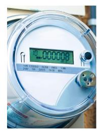
For many years, electric meters have been the sole responsibility of electric utilities. Building owners are now installing their own electric meters to determine the power produced by on-site renewable energy sources, such as solar or wind. Green construction codes require a means for measuring, monitoring and reporting on energy use, production and reclamation in a building, which is accomplished by smart meters.
